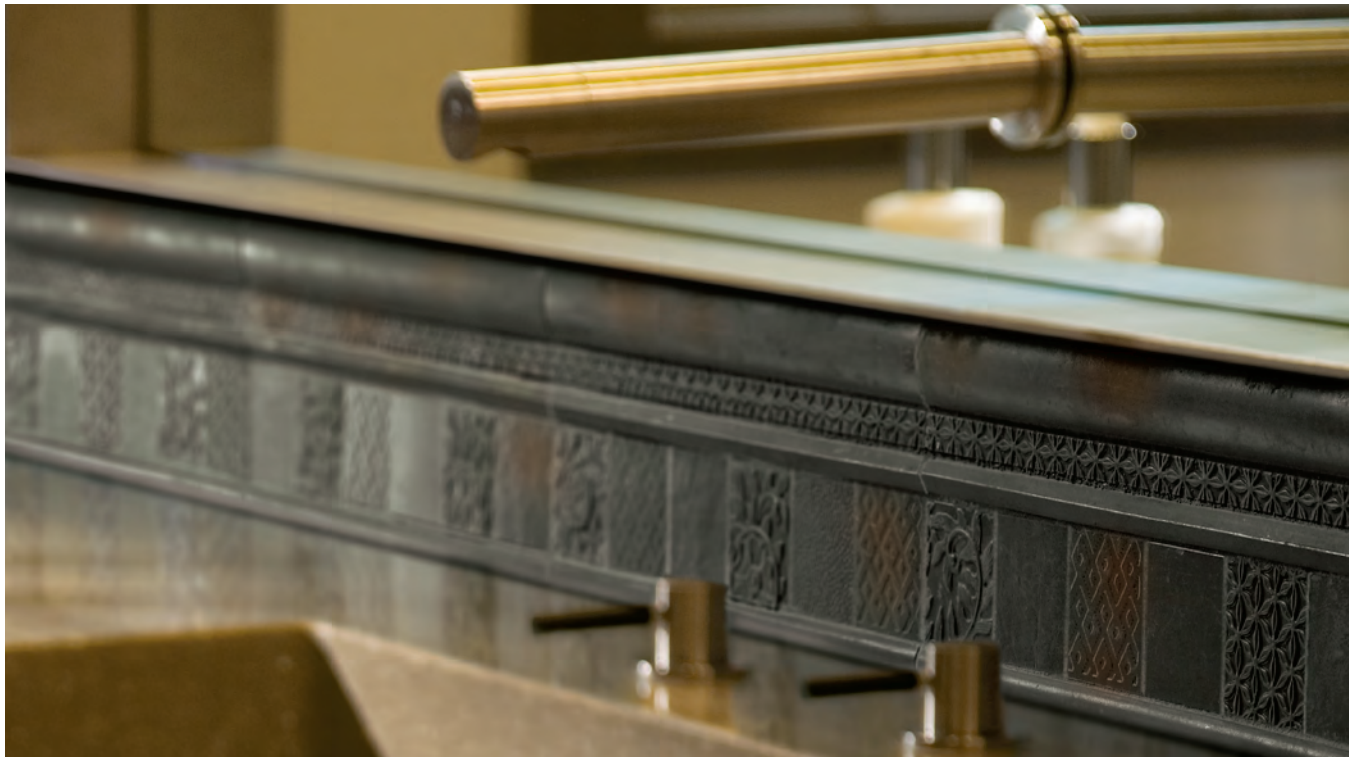
Products featured in photo above: Iron Nickel Variegated – 1-1/4" x 12" Dome Liner, 1/2" x 12" Starflower Liner, 1/2" x 12" Arrowhead Liner, 4" x 12" Mosaic Border (1 row of 2' x 2'), 1/2" x 12" Pencil Liner
